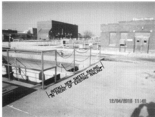
2 PHOTOGRAPH - TYPICAL CONDITIONS PRELIMINARY SETTLING TANKS - INSTALL NEW SAFETY RAILING IN FRONT OF EXISTING
