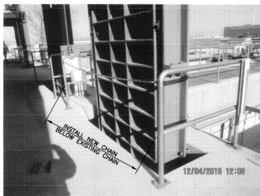
10 PHOTOGRAPH - TYPICAL CONDITIONS PRELIMINARY SETTLING TANKS - INSTALL LOWER CHAIN SEE DETAIL DRAWING S-201
