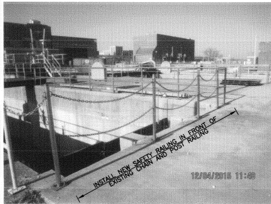
1 PHOTOGRAPH - TYPICAL CONDITIONS PRELIMINARY SETTLING TANKS - INSTALL NEW SAFETY RAILING IN FRONT OF EXISTING
