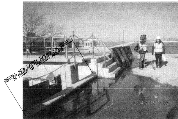
4 PHOTOGRAPH - TYPICAL CONDITIONS PRELIMINARY SETTLING TANKS - INSTALL NEW SAFETY RAILING ON CURB
